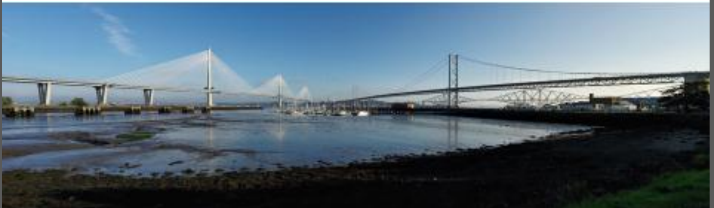
Queensferry Crossing Scotland
