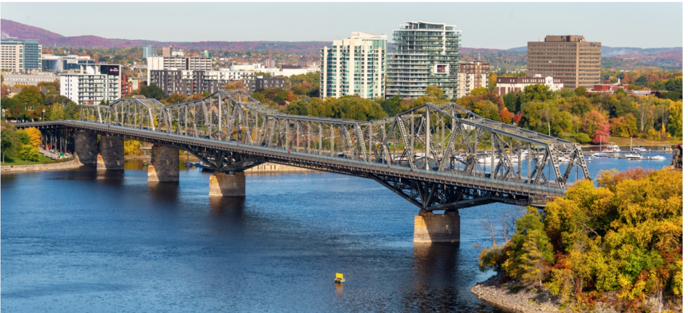
Figure 1: The Alexandra Bridge, Ottawa, Ontario. Source: Architects DCA Inc.
