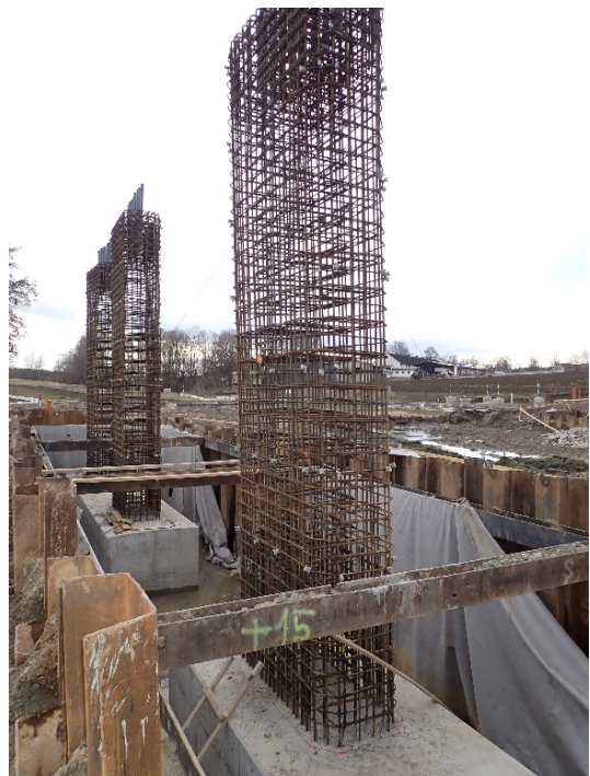
Figure 8: Reinforcement of the foundations and piers on the construction site
