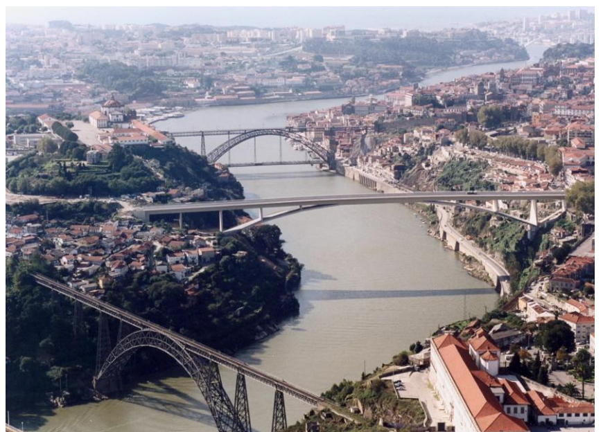
The Infante Don Enrique laminar arch bridge, Porto, Portugal
