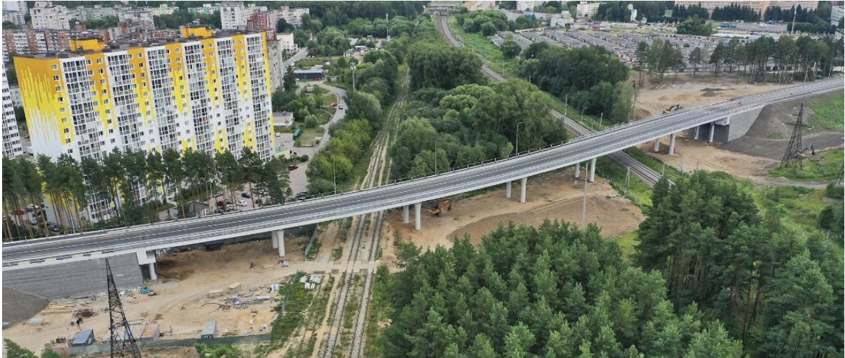
Figure 5: The overpass after the construction work was completed
