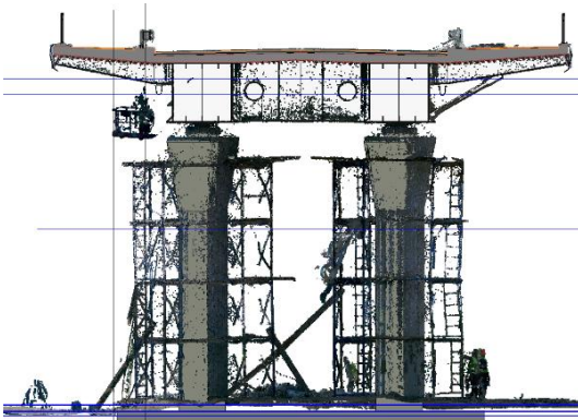
Figure 10: Control of geometric parameters of the span structure and pier in the section of intermediate pier No. 6. Green values represent low deviations (low distances) between the cloud and the model, while red or blue indicates large differences
