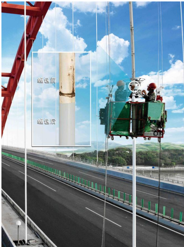
Figure 5: Special maintenance of the cable system
