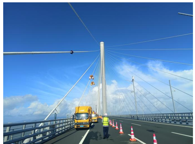
Figures 7 and 8: Bridge cable inspection using a climbing robot
