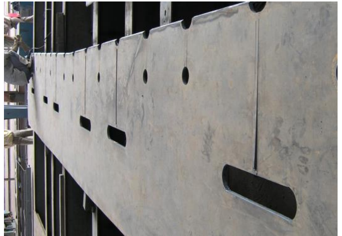
Figure 20: The cross beam web the approach bridge
