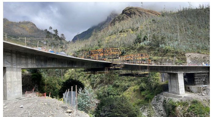
Figure 9: Construction of Ollachea Bridge 2, Perú
