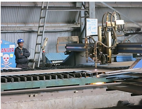
Figure 22: Web plate cutting by NC-machine
