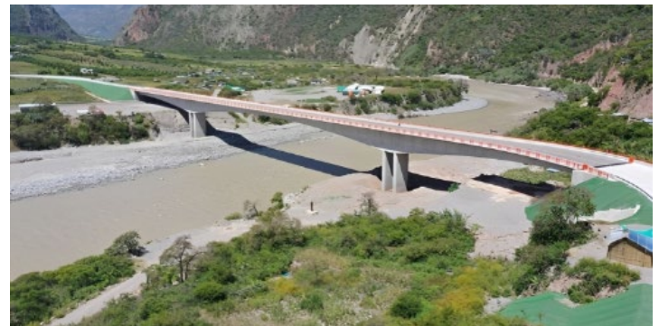
Figure 16: Pampas Bridge, Ayacucho, Perú
