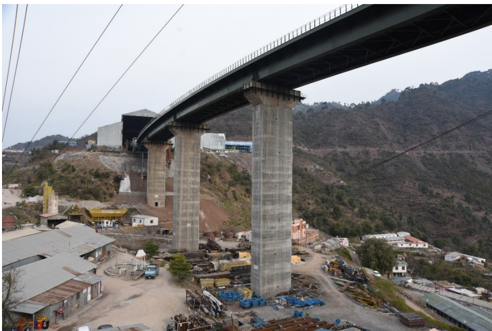
Figure 7: Approach Viaduct with the fabrication facilities on the background
