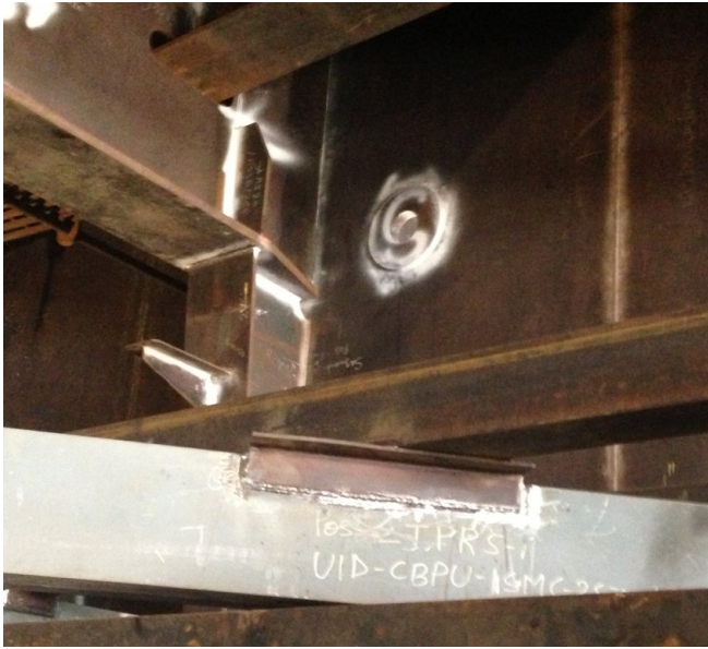
Figure 8: The reinforced web hole for the turning rod of the segment
